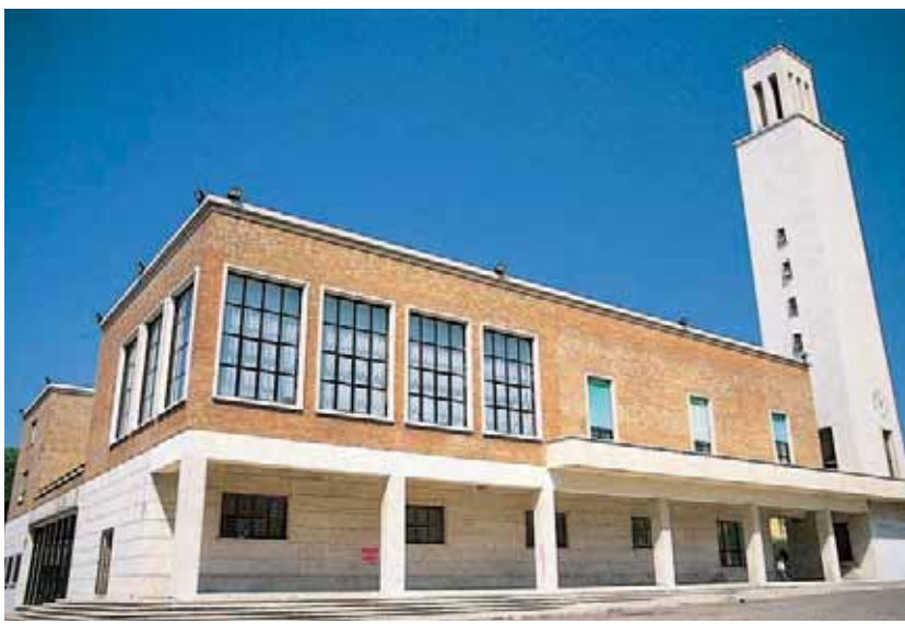
Above, the Town Hall, with the 42-metre civic tower.
